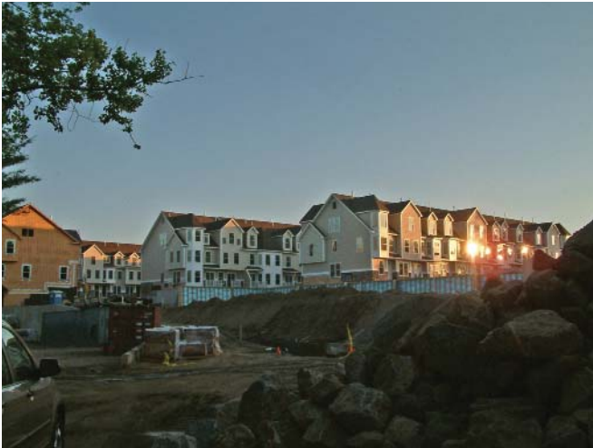
Figure viii. Housing under construction in Stamford, CT
